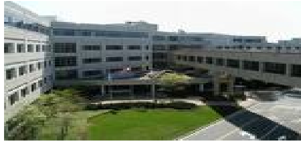
Washington Hospital Center
